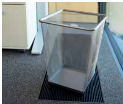
Fig. 2: Blocked air outlet.
